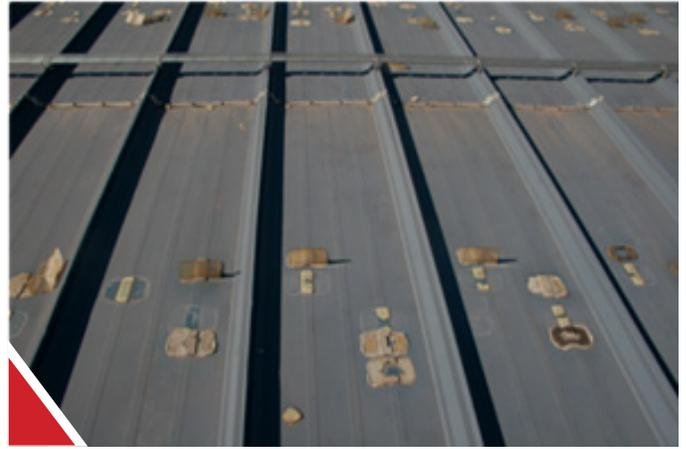
Adhesive attached snow retention devices are often prone to failure and can damage the coating system and void coating and substrate warranties.
