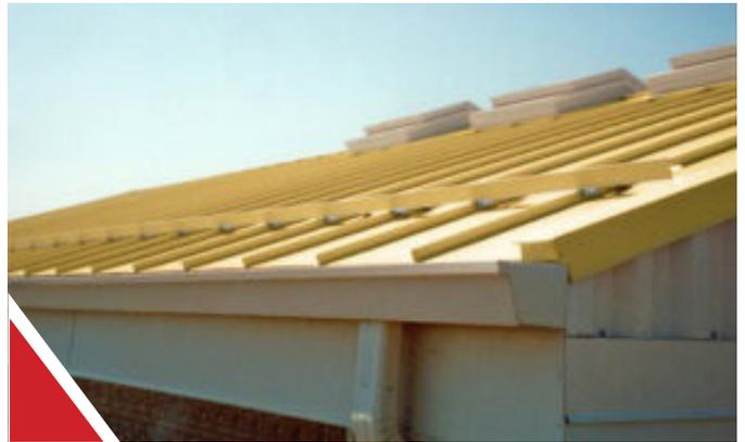
S-5! ColorGard system utilizes clips that attach to standing seams without adhesives or penetrating the roof systems.
