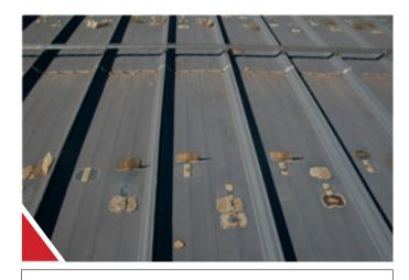
Adhesive attached show retention devices are often prone to failure and can damage the coating system and void coating and substrate warranties.
