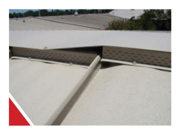
only when they are properly installed. When panels get off-module during installation (meaning they grow or shrink from the intended panel width) it can be challenging to make the system watertight.
