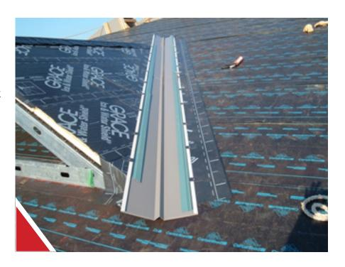
diverters as steep as possible but a minimum of 1½" high; include backup water protection such as ice and water; require shop drawing of proposed detail and require valley trim with integral cleats as shown in photo above.
