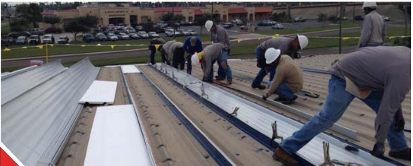
Using multi-span clips can triple the wind uplift capacity without removing the original roofing system. Consequently, this approach dramatically reduces labor, material cost and disruption to occupants and business operations.
