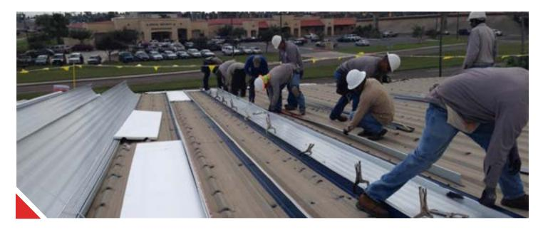
Using multi-span clips can triple the wind uplift capacity without removing the original roofing system. Consequently, this approach dramatically reduces labor, material cost and disruption to occupants and business operations.
