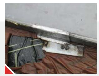
This photo shows an example of a two-piece asymmetrical standing seam panel clip destroyed by excessive thermal movement of the roof panels. The panels were too long for the clip.
