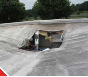
These two images show the potential risk of installing a single-ply roof over a metal building roof. Fortunately, no one was in the building when the roof collapsed.
