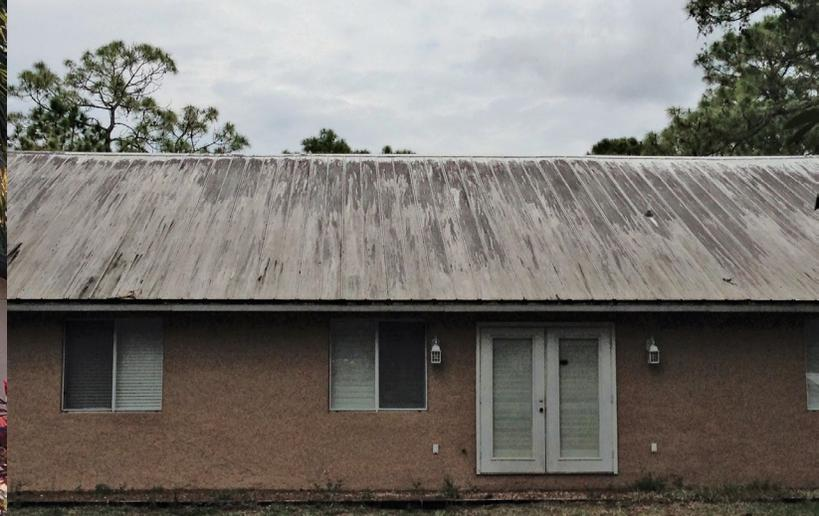
Picking a quality metal roof and using a reputable contractor to install it is important. Above right, an inferior metal roof with a sub-quality paint system grew fungus. The homeowners replaced it with a Drexel Metals roof in Mansard Brown (above left).
