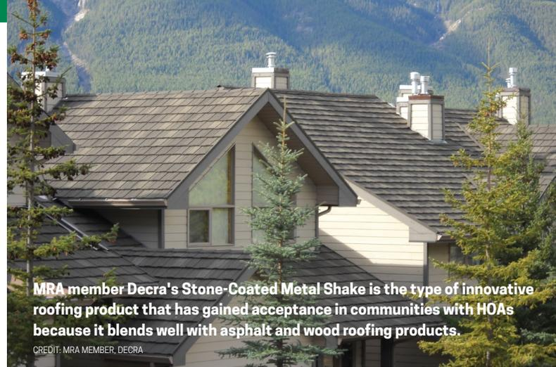
**MRA member Decra's Stone-Coated Metal Shake is the type of innovative roofing product that has gained acceptance in communities with HOAs because it blends well with asphalt and wood roofing products.**
