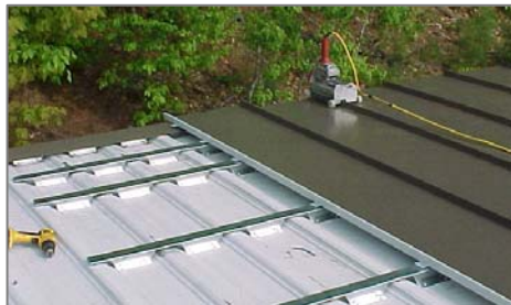
Courtesy of Roof Hugger®, Inc.
