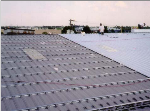
Courtesy of Roof Hugger®, Inc.
