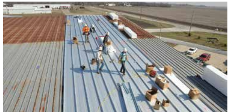
Single length panels offer labor savings and improve weathertightness.
