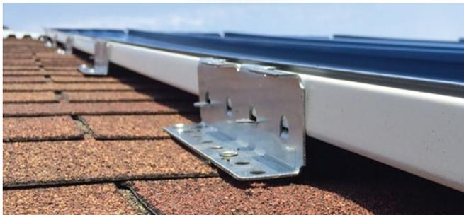
The key to proper installation of standing seam recover over shingles is the patented shingle recover clip, which is long enough to sit on two shingles simultaneously
