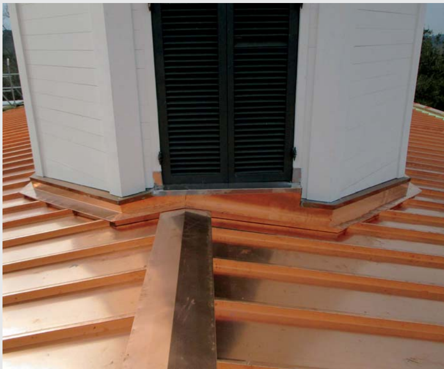
Standing seams were incorporated at each hip of the cupola. At the apex of the cupola, the seams were folded down and lapped under the finial skirt.
