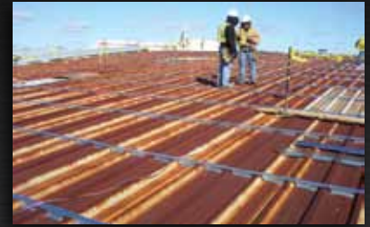
Roof Hugger installation
