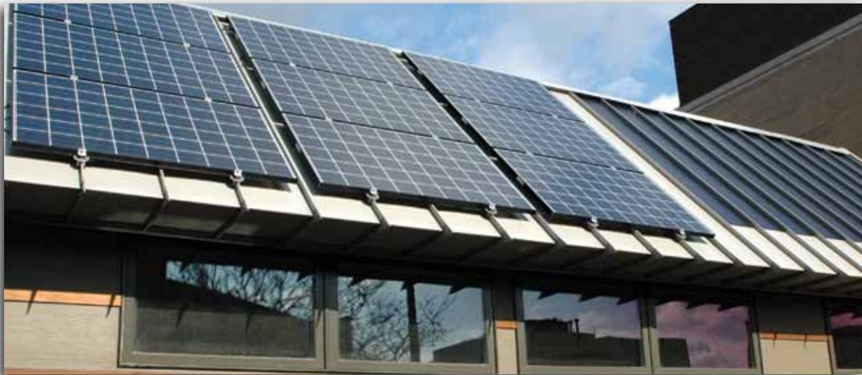
Example of crystalline photovoltaic panels (left) and thin-film panels (right)
